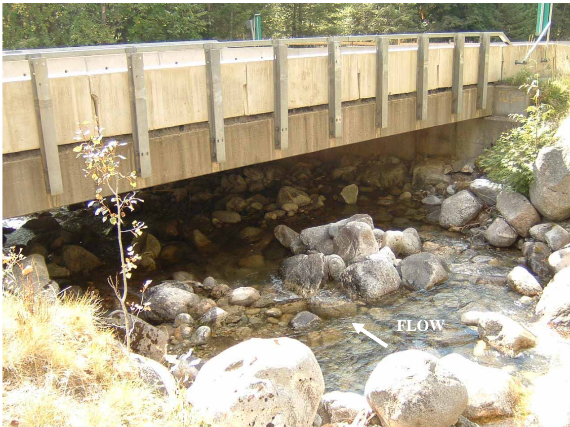
Photo 2 Upstream side of Highway 3A bridge (September 12, 2007)
